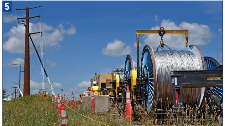
materials that do not allow electricity to pass through them. Trucks, heavy equipment and sometimes helicopters, are used to string the lines. Other equipment, including bird diverters, spacers and devices to prevent the wires from galloping (moving up and down during icy, windy weather conditions) may also be installed.
